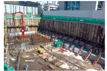
Concreting of Raft Foundation by Auramix 300
