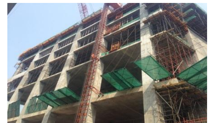
Construction of Tower A till Sep'14
