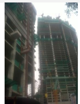
Construction of Tower B till Sep'14
